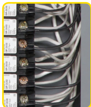
▲ Pigtail Neutral connection
