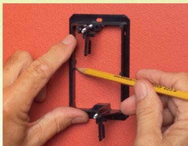
Locate bracket position. Level. Trace inside of LV1 and cut on the outside of the line.
