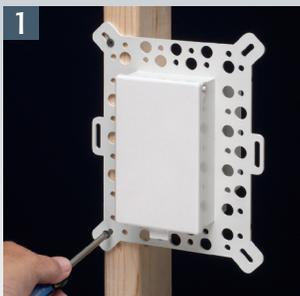
1 Install NM cable connector and wire. Attach IN BOX to stud.
