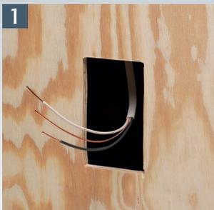
1 Make a 3-1/4" x 5-1/2" hole in plywood. Pull wiring through opening.
