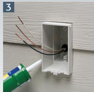
3 Cut rigid siding to fit around IN BOX. Caulk around box.
