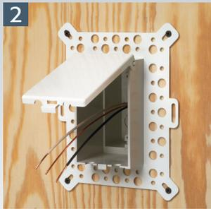
2 Install NM cable connector and wire. Attach recessed IN BOX to plywood.
