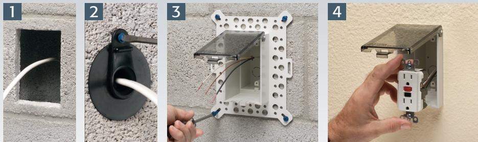
1. Make a 3-1/4" x 5-1/2" hole in block. Pull wiring through plastic block bushing and opening in block. Block bushing mounts to interior side of block.
