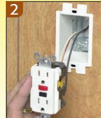
2 Attach wires to receptacle. Then tighten screws for a level, fully supported, code compliant installation.
