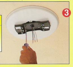
Install the fixture or fan mounting bar (provided with fixture or fan) directly to the joist with the (2) #10 x 3" wood screws and lock washers provided.
