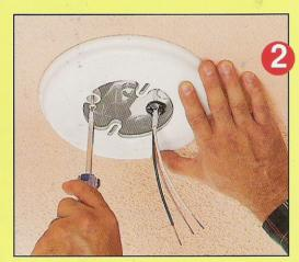
Using the #8 x 1-1/2" wood screws (provided), mount the MB8 to the joist (through the ceiling).
